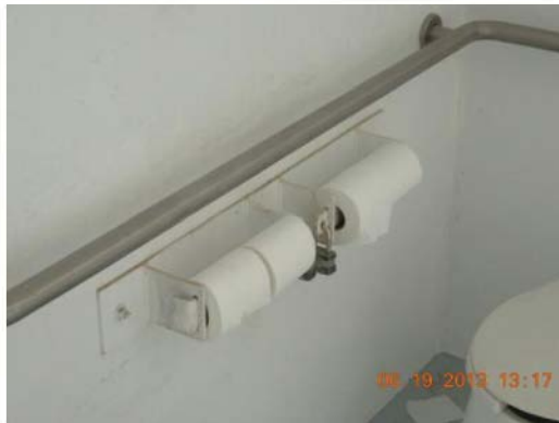
Stocked toilet paper bars in vault toilet
