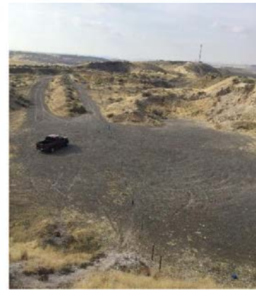
Pasadena Gravel Pit fence
