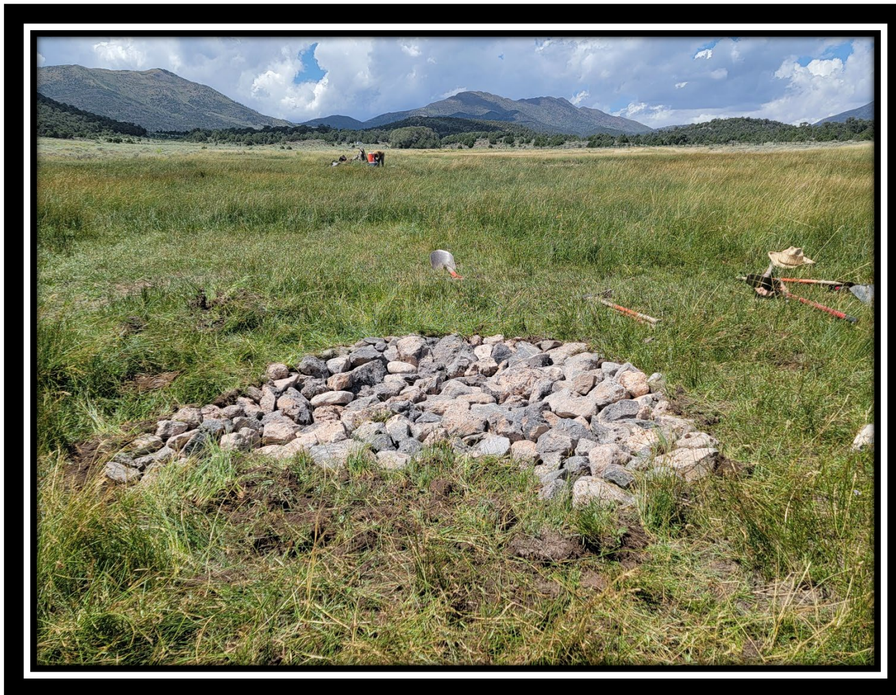
Photo (After): Rock Layback Structure
