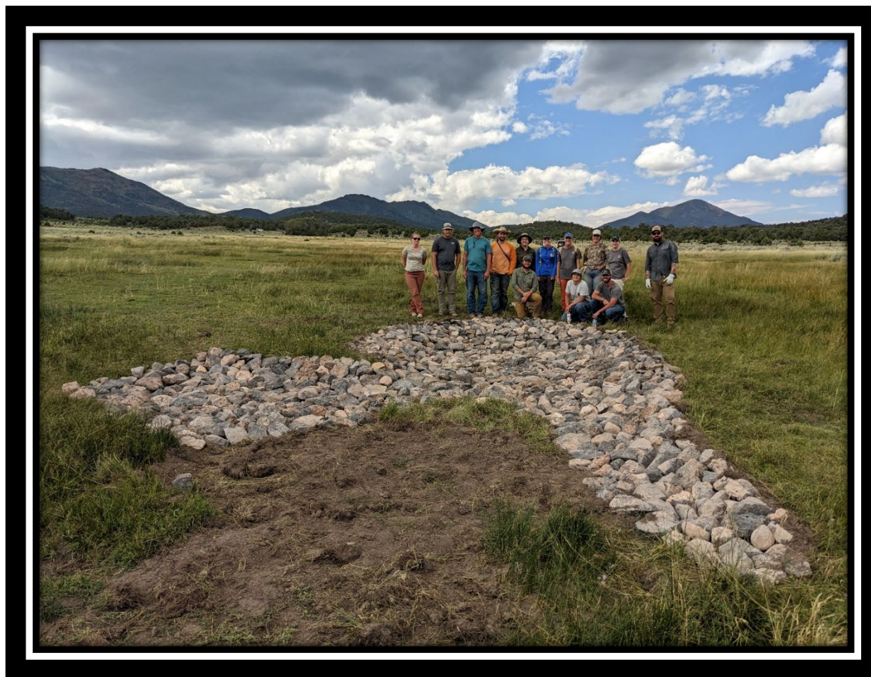
Photo (After): Rock Layback Structure
