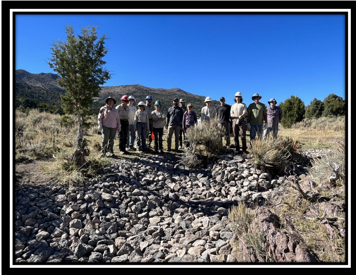
Photo (After): Rock Layback and Zuni Bowl Structure
