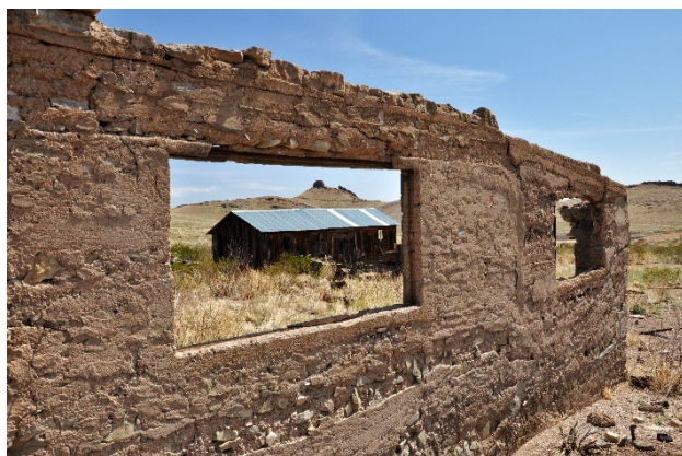
Figure 18: A view of the buildings at Lake Valley.
