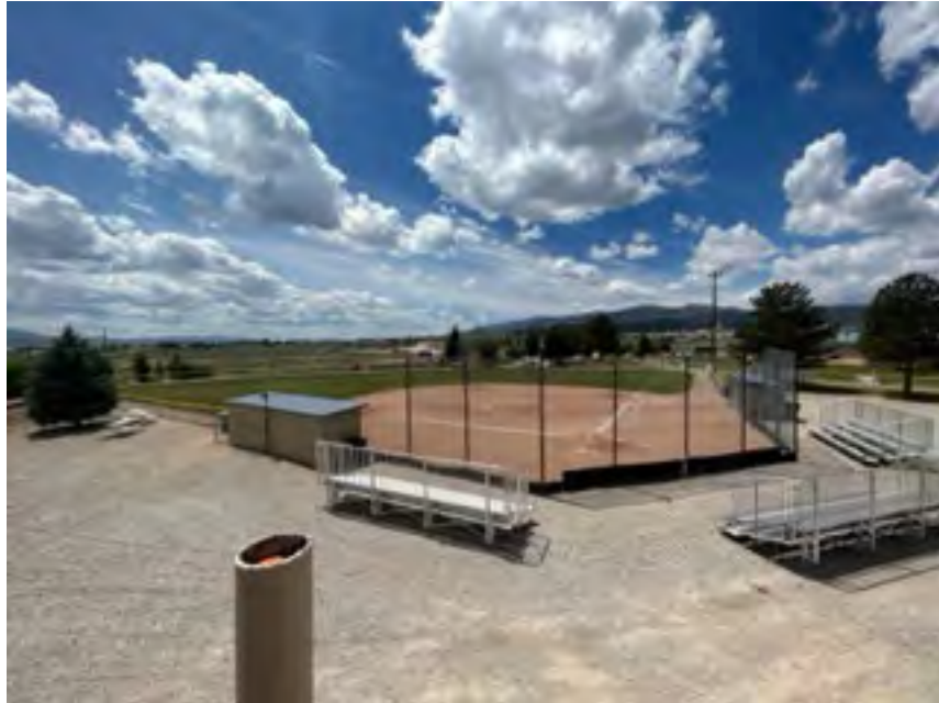
Photo 1: Ely Little League Fields Renovation Field 2 from Press box, Looking Southwest
