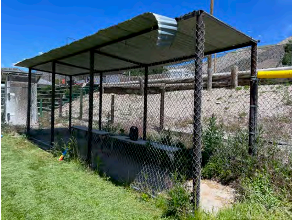
Photo 3: Little League Field Dugout and Sprinkler/Maintenance Shed
