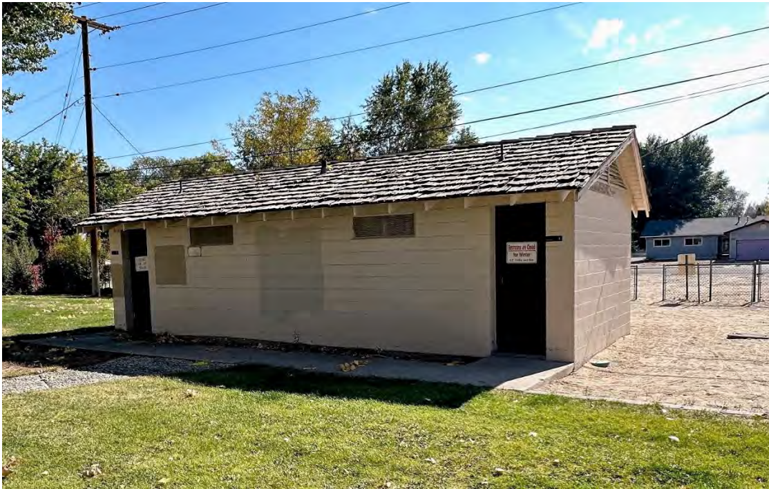
Photo 5 – Restroom at west end of Mills Park will be replaced.
