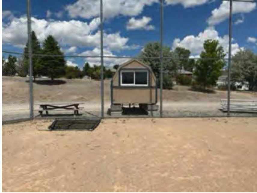
Photo 3: Ely Little League Fields Renovation-Field 2 Press box from home plate looking North
