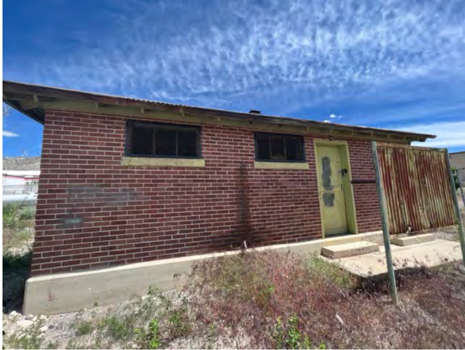
Photo 5: Original Restroom Building
