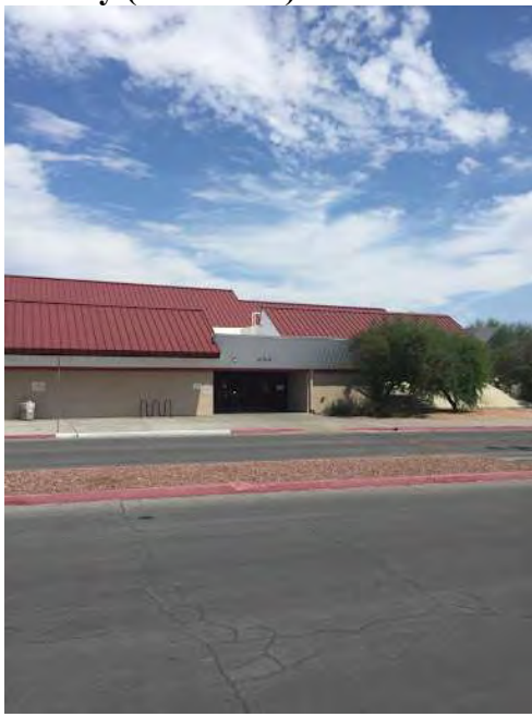
Facility (south side)
