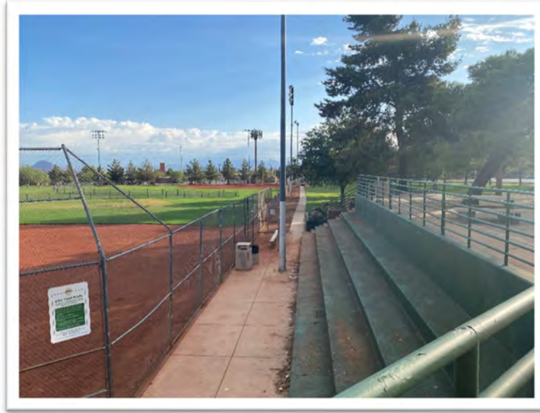
Photo 5: Project site view of the baseball fields seating area. Taken at the southeast corner of the baseball fields complex and looking north-east across the baseball fields, with distant views of the surrounding mountains, it highlights limited natural surveillance.
