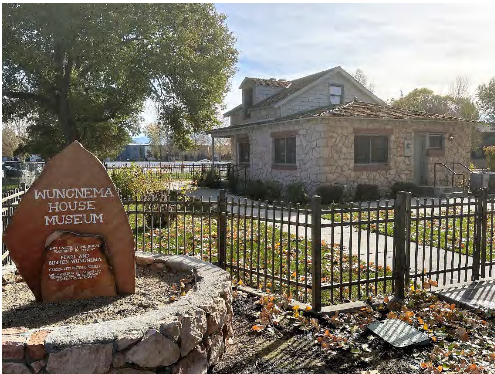
Photo 4 – Historic Wungnema House. Improvements will be implemented per 2021 Carson City Facilities Assessment.
