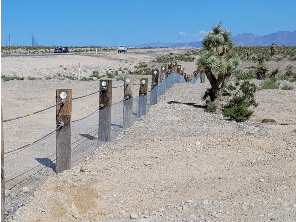
Photo 3: Example post-and-cable tortoise fence
