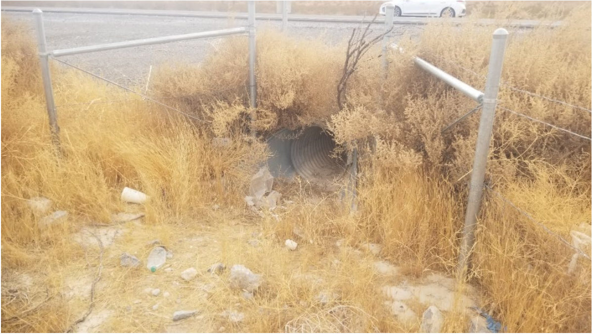
Photo 3. Corrugated metal culvert with fencing attached.
