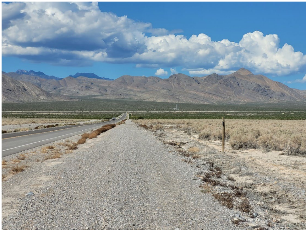
Photo 2: Corn Creek Road West
