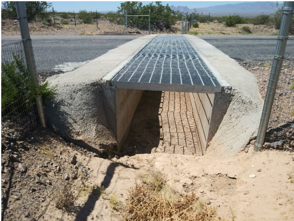
Photo 6: Wildlife culvert example
