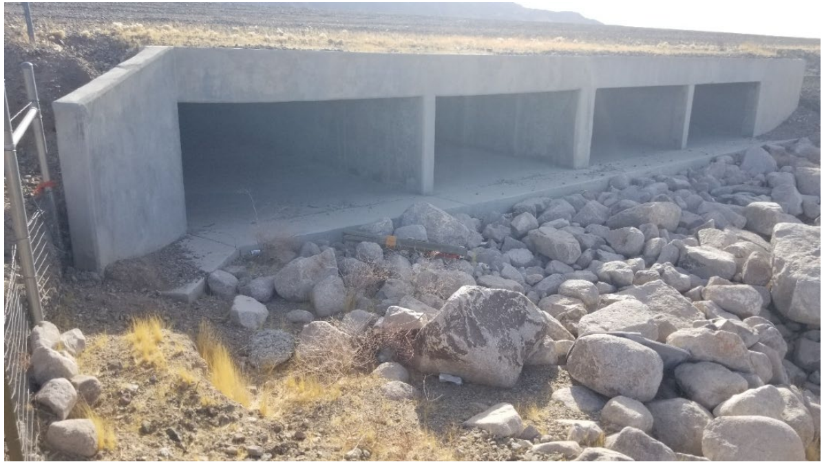
Photo 4. A large concrete box culvert with fence attached.
