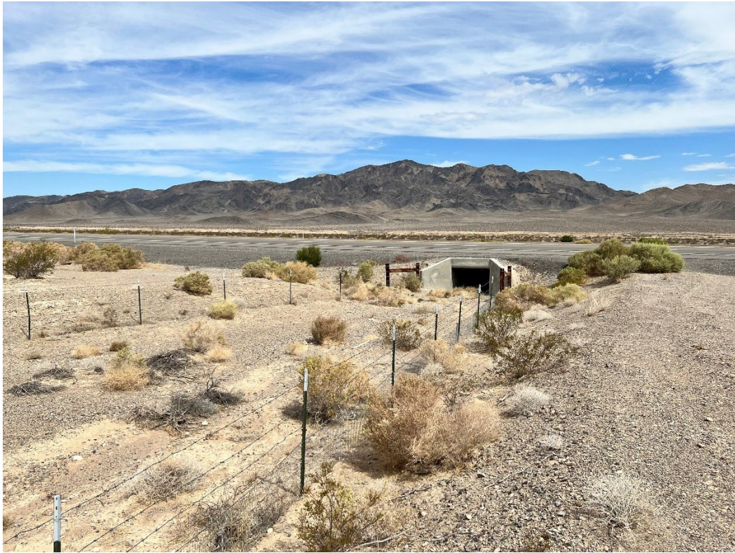
Photo 1. Small concrete box culvert with desert tortoise fencing attached.
