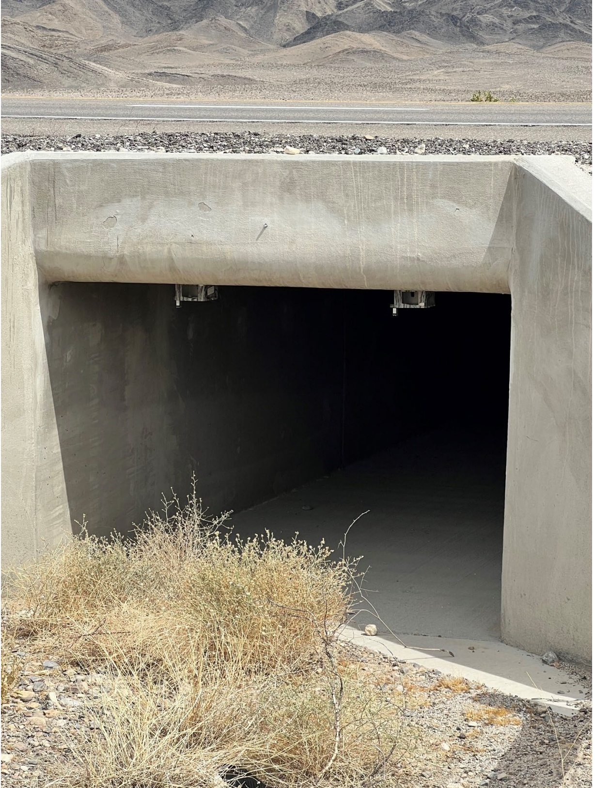
Photo 5. This photo depicts how cameras will be placed inside the culverts.
