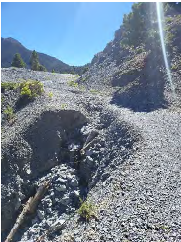
Photo 5: Example of erosion damage along lower portion of the trail.
