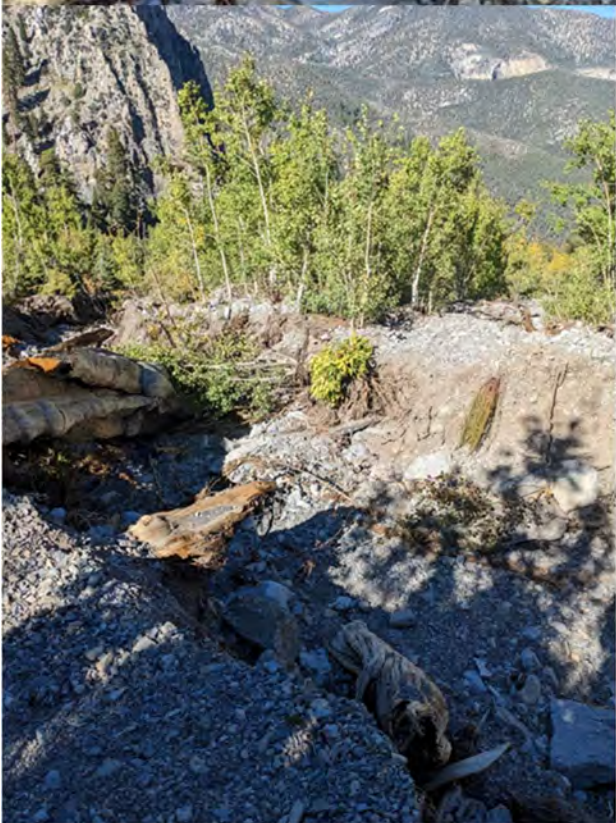
Photo 3: Significant trail damage (complete loss of trailway) at trail mile 0.9.
