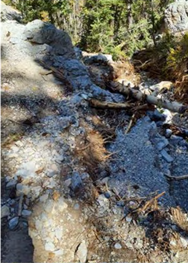
Photo 3: Example of complete washout and loss of trailway found post-damage on the upper portion of the Bristlecone Trail.
