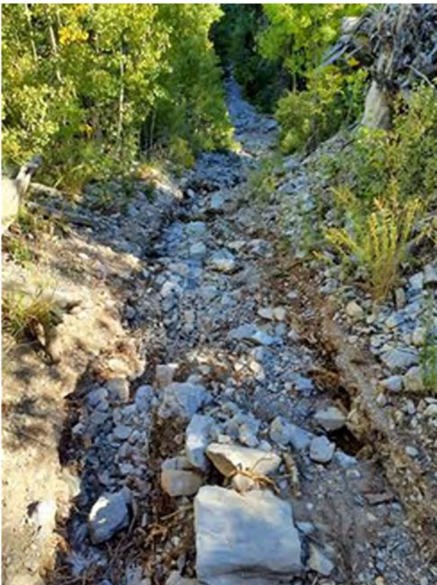
Photo 2: Typical trail damage between trail mile 0.2 and 0.9.
