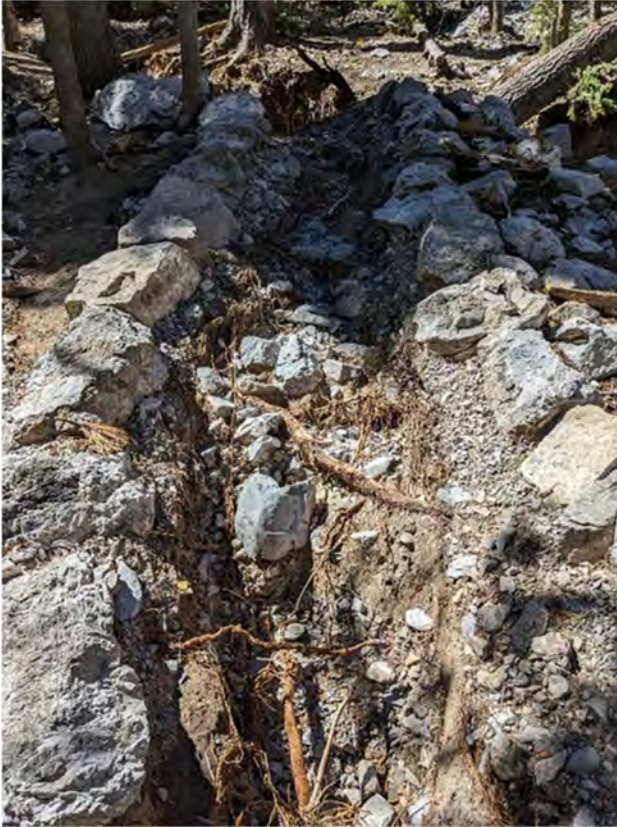
Photo 1: Typical example of severe rutting along trailway on upper portion of the trail.
