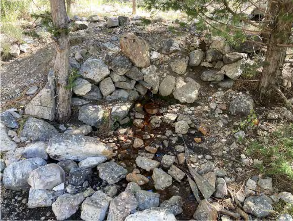
Figure 6: Wiregrass Spring, unreliable and in need of complete refurbishment to provide reliable water source with wildlife drinker.
