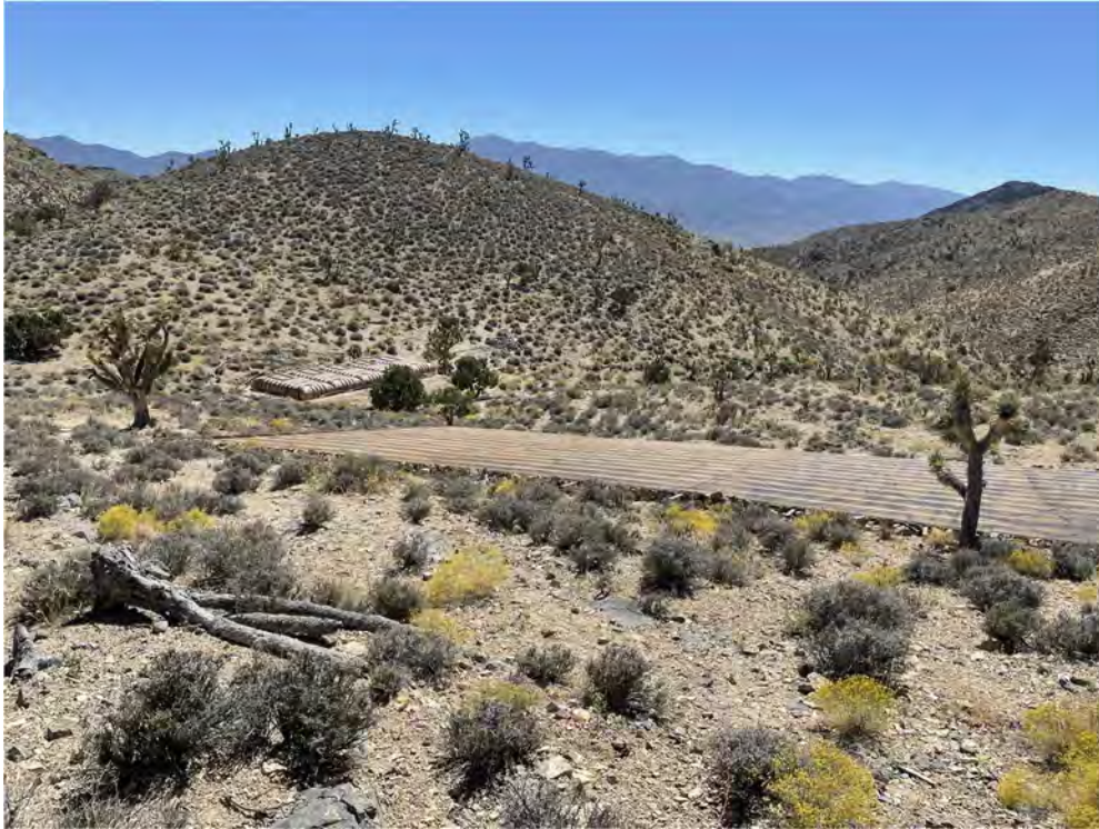
Figure 1: Example of newly rebuilt guzzler with new, camouflaged metal apron in the foreground and new camouflaged flat storage tanks and self-leveling drinker in the background. This Saddle Mountain guzzler rebuild was funded by SNPLMA Rd. 19
