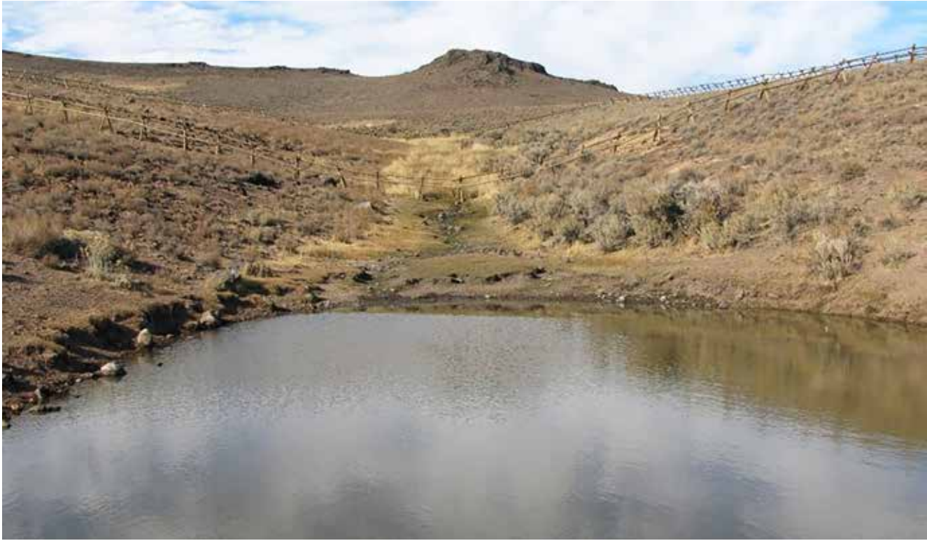
Figure E4. Artificial stock pond constructed for livestock water. This structure was specifically designed as a livestock watering facility and, because the pond source is a combination of surface runoff and limited seasonal groundwater discharge, it has little potential to develop riparian or wetland attributes. There is a small livestock concentration zone in the vegetated drainageway between the fence and the pond. However, this small, localized impact zone is to be expected at this site. Because this pond is a designed watering facility and has little potential for developing riparian or wetland attributes, monitoring would not be recommended at this site. However, a reference plot may be installed inside the enclosure if desired to monitor the condition of the seasonally wet vegetated drainageway (provided that it meets the applicable ecosystem criteria in the Section 1.2 criteria box).
