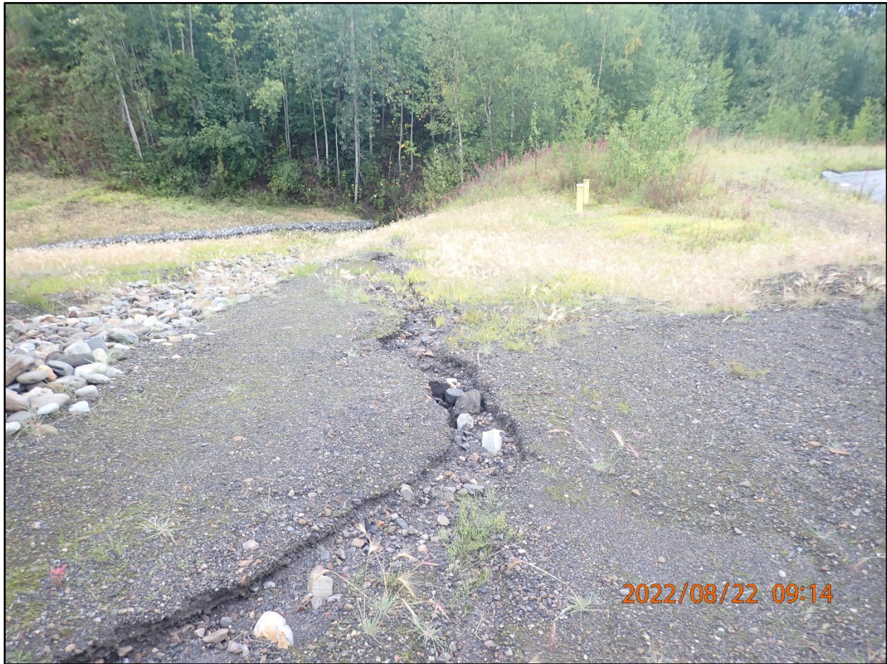
Photograph 2-6. Erosion features adjacent to MW16 and MW17, August 2022.
