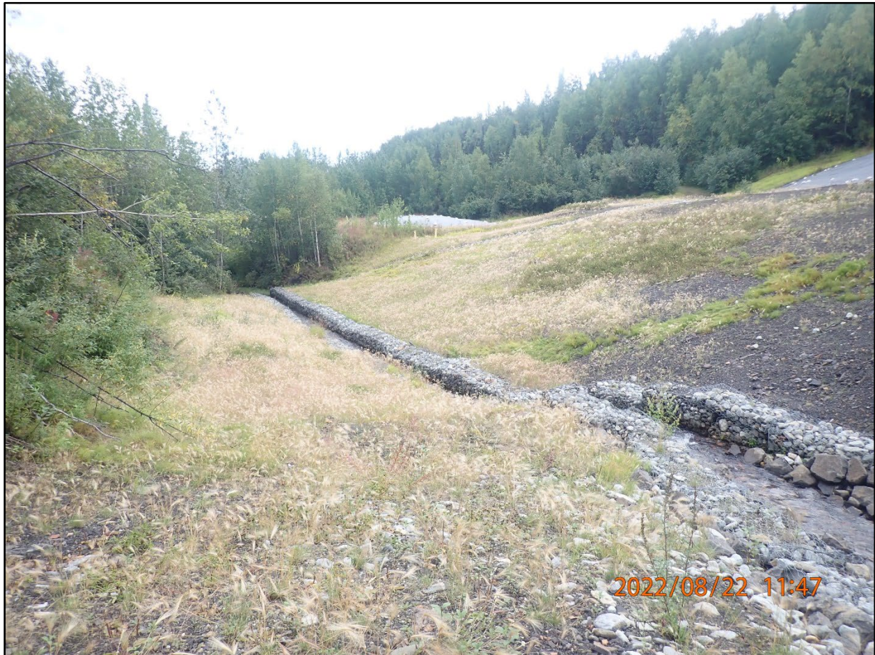
Photograph 2-8. Reworked Red Devil Creek stream channel with gabions, August 2022.
