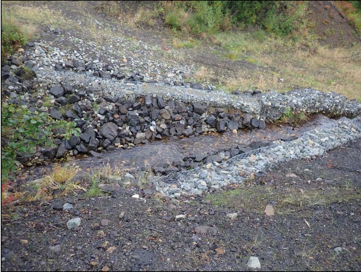
Photograph 2-27. Red Devil Creek reworked section with gabions. September 2, 2021.
