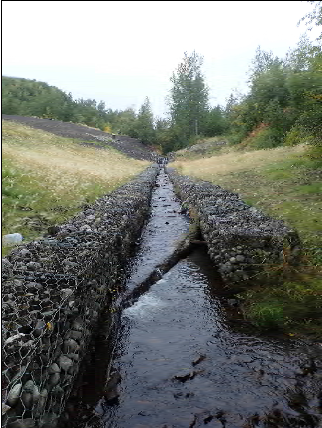
Photograph 2-28. Red Devil Creek reworked gabion section, looking upstream. September 2, 2021.
