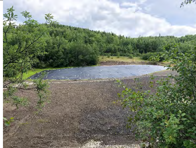
Date: 6/23/2020 Direction: SW Description: Damaged ropes and sandbags located on monofill.
