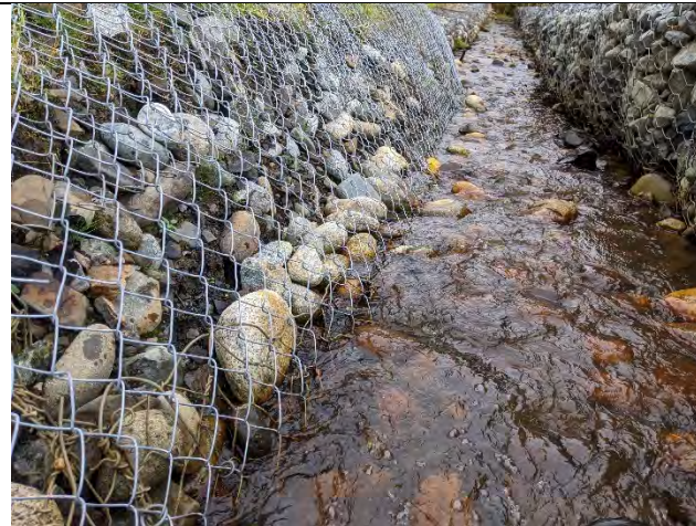
Date: 9/9/2020 Direction: NE Description: View of repairs made to damaged gabions.
