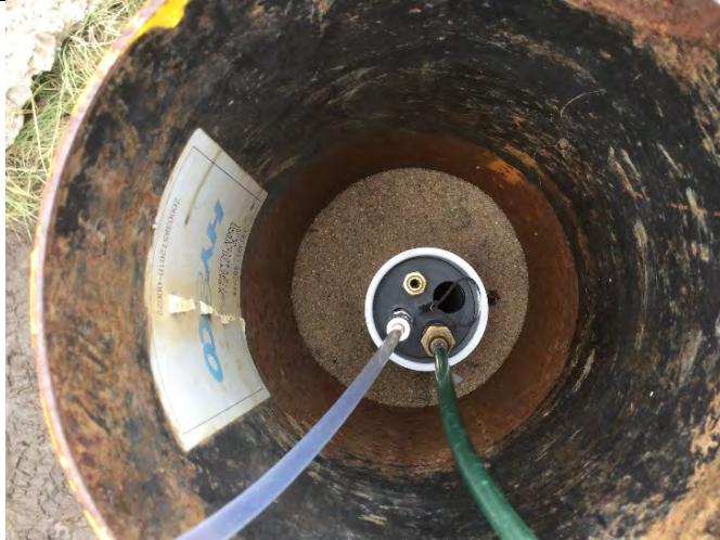
Date: 9/3/2020 Direction: Down Description: Dedicated well cap installed in MW10.
