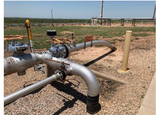
Crude Helium 8" Pipeline at Cliffside
