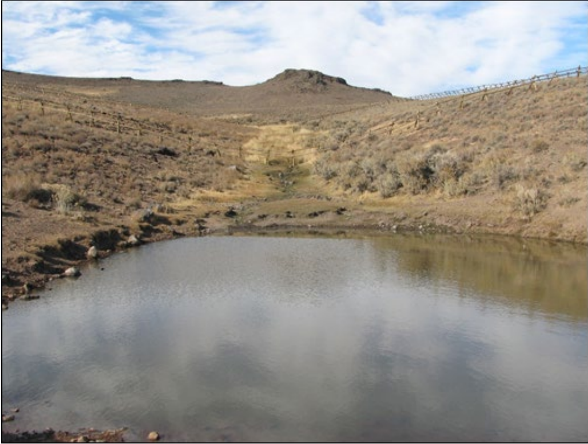
Figure E4. Artificial stock pond constructed for livestock water. This structure was specifically designed as a livestock watering facility and, because the pond source is a combination of surface runoff and limited seasonal groundwater discharge, it has little potential to develop riparian or wetland attributes. There is a small livestock concentration zone in the vegetated drainageway between the fence and the pond. However, this small, localized impact zone is to be expected at this site. Because this pond is a designed watering facility and has little potential for developing riparian or wetland attributes, monitoring would not be recommended at this site. However, a reference plot may be installed inside the enclosure if desired to monitor the condition of the seasonally wet vegetated drainageway (provided that it meets the applicable ecosystem criteria in the Section 1.2 criteria box).
