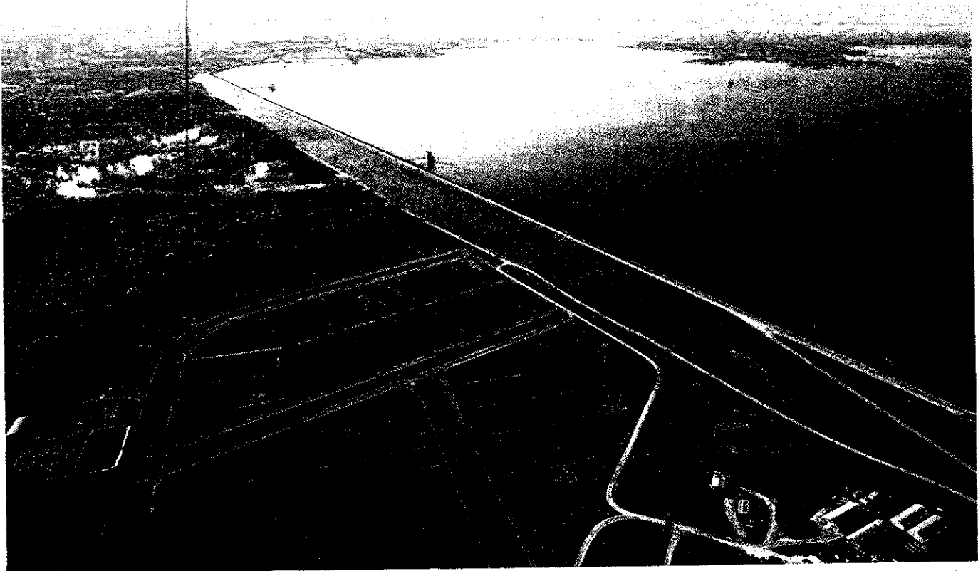
Only 34 miles upstream from Dallas , the 6.2-mile-long Lewisville Dam holds back 2.5 billion tons of water when the lake is full. That's 125 times as much as the dam that failed in Johnstown, Pa., in 1889, killing 2,209 people in the nation's worst flood.
