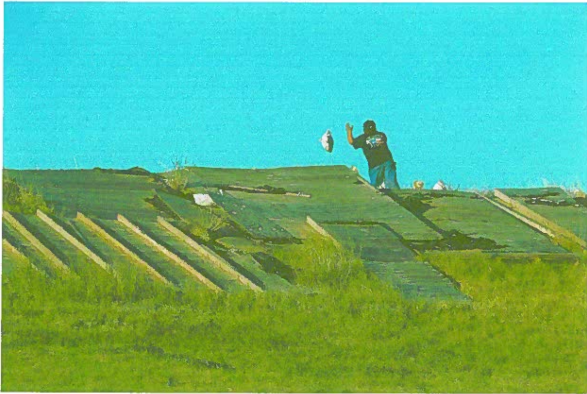
Workers throw sandbags and lay tarps to prevent further erosion of the slide on the dam. Corps of Engineers officials say a more permanent fix would cost between $50 million and $500 million.
