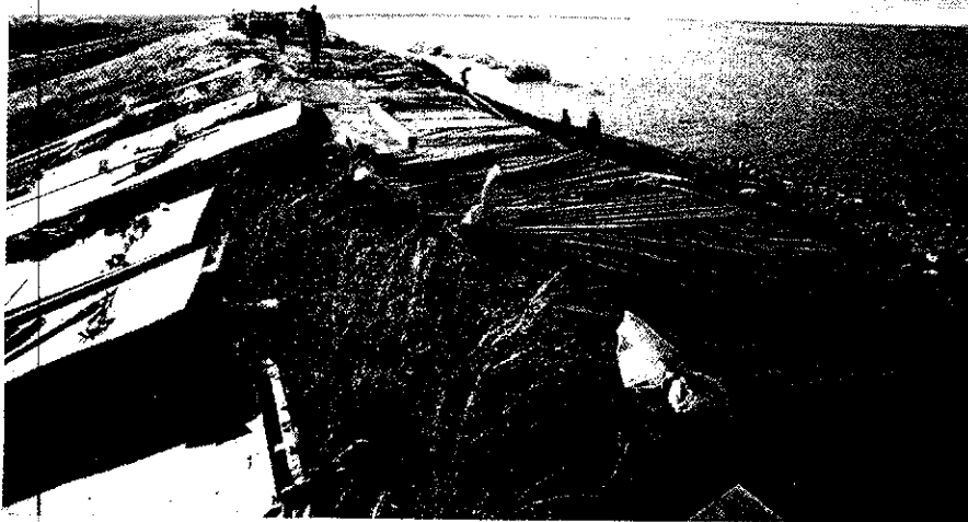
Workers deploy sandbags and tarps to temporarily prevent further erosion along a 160-foot-long slide in the Lewisville Dam. Corps engineers say the embankment is more unstable since the May flood because cracks have spread along the 20-foot-wide crest of the dam.
