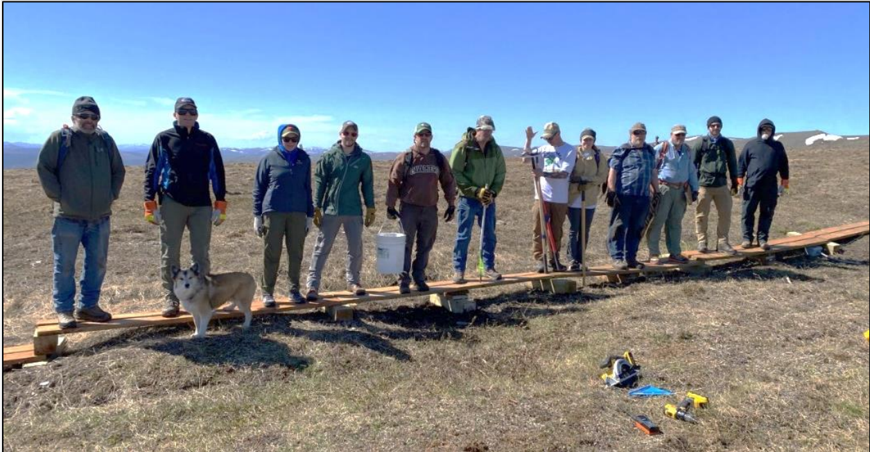
Figure 9. Volunteers test the strength of the boardwalk after reinforcing it.
