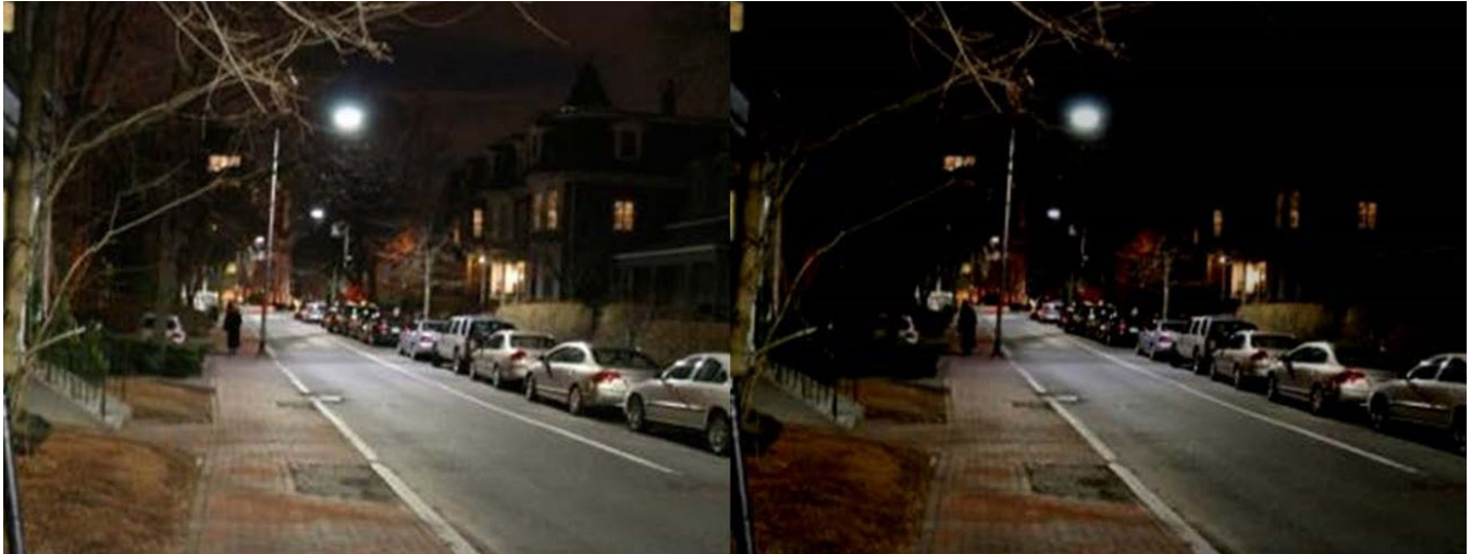
LED street lighting system shown at initial startup at dusk (left) and 50 percent dimmed after midnight (right).
