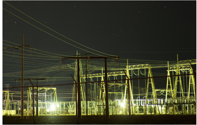
Unshielded lighting at this electrical substation in Nevada is a major source of light trespass and glare into the surrounding desert.
