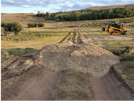
Photo during construction process.
