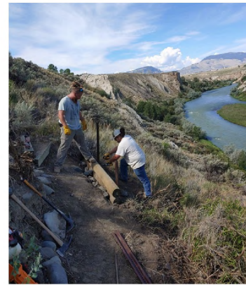
BLM seasonals building a retaining wall on Seven Mountain Trail
