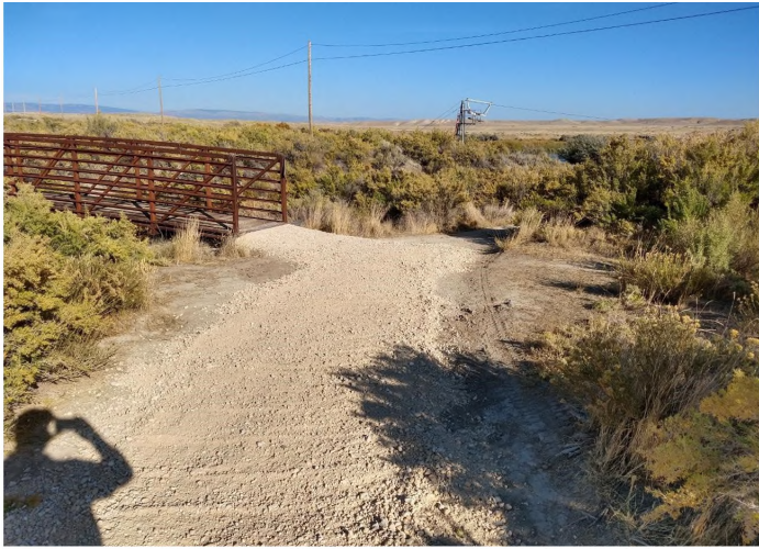
Continuing trail improvements at Blue Gulch.
