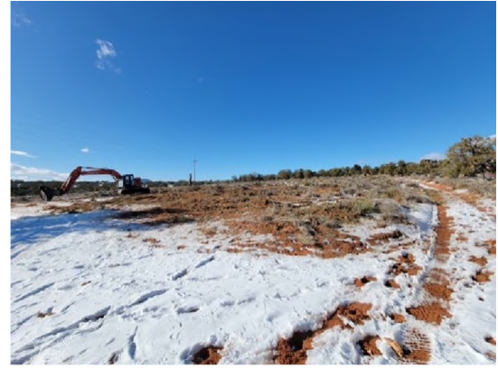
Machine Performing Vegetation Clearing
