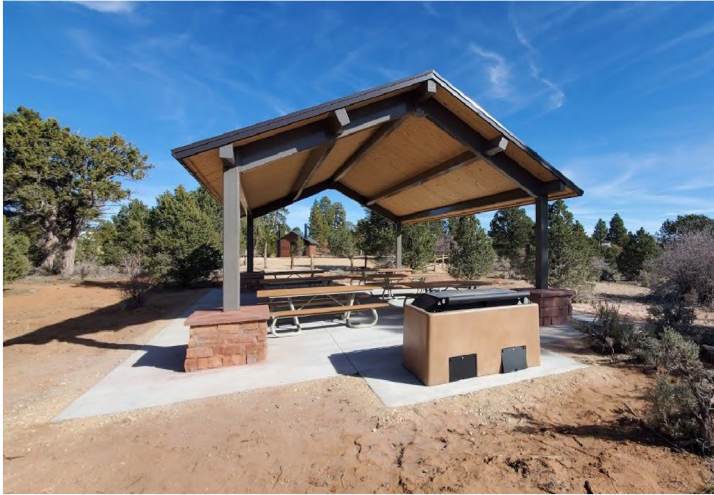
Add Gravel To Apron At Group Sites
