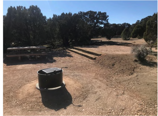
Newly-installed Fire Ring at Rocky Peak Campground
