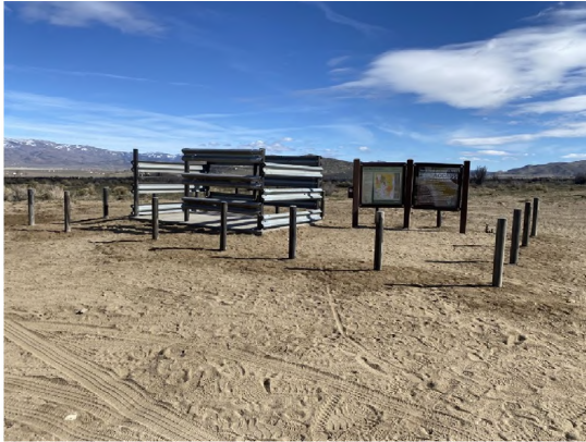
Newly Completed Portable Restroom Pad.
