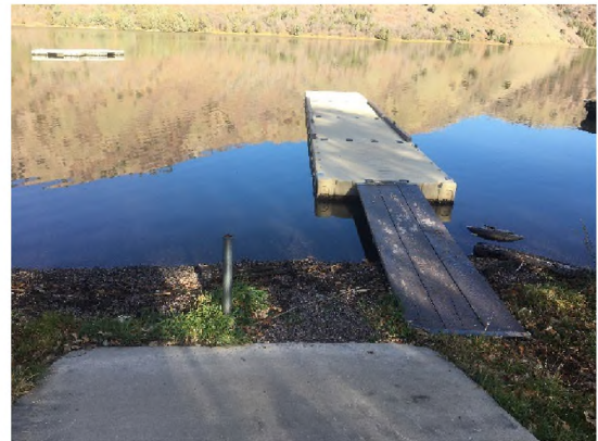
Installing new gangway at Maple Grove Campground
