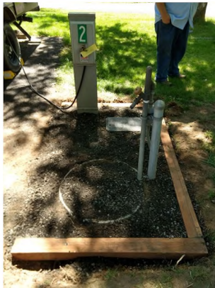
Improvements to Hydrant and Electrical Posts
