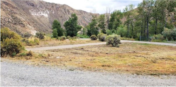
Ground work of Bayhorse campsite expansion
