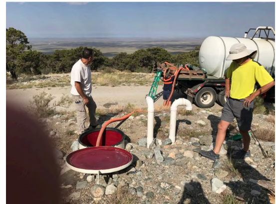
Camp Host Site Potable Water
