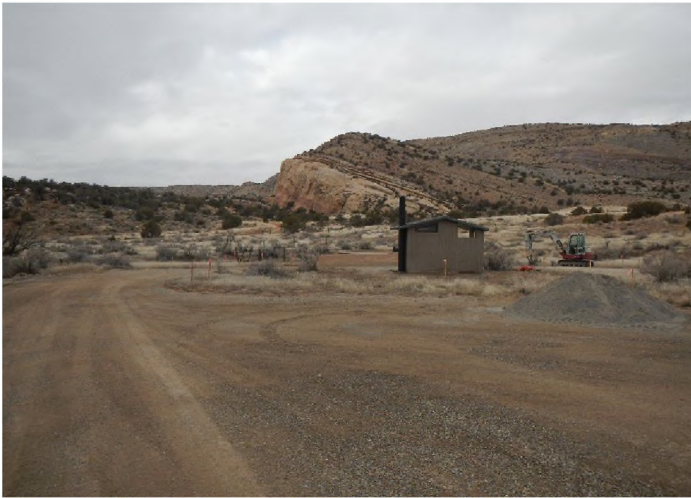
Construction on the Equestrian Campground
