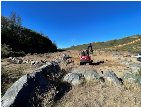
B. Berry Runs Excavator at Westside Staging Area
