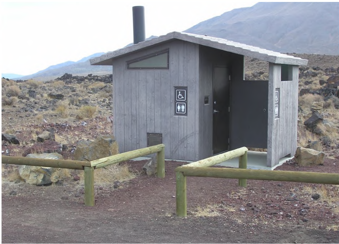
Fossil Falls Campground Accessible Vault Toilet
