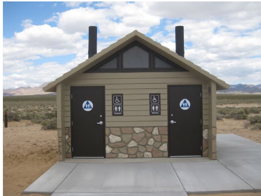
Ivanpah Dry Lake vault
