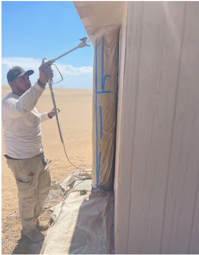
Maintenance staff painting a CXT vault toilet.
