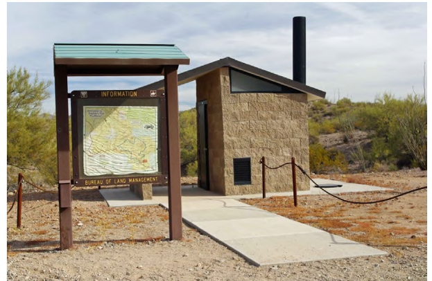
Vault Toilet at Sophie's Flat
