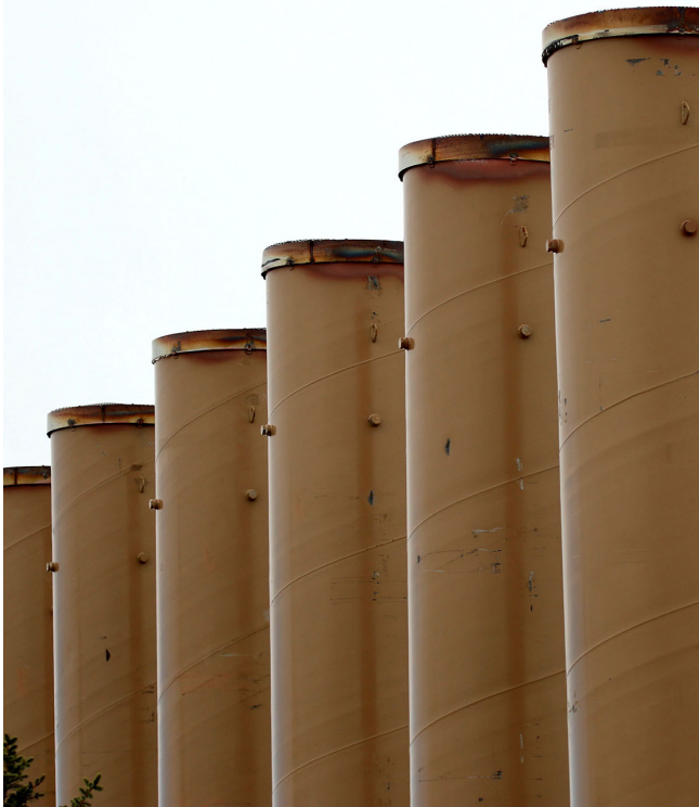
Enclosed flare systems have no visible flame, and their use minimizes ecological and aesthetic effects, while reducing emissions.
