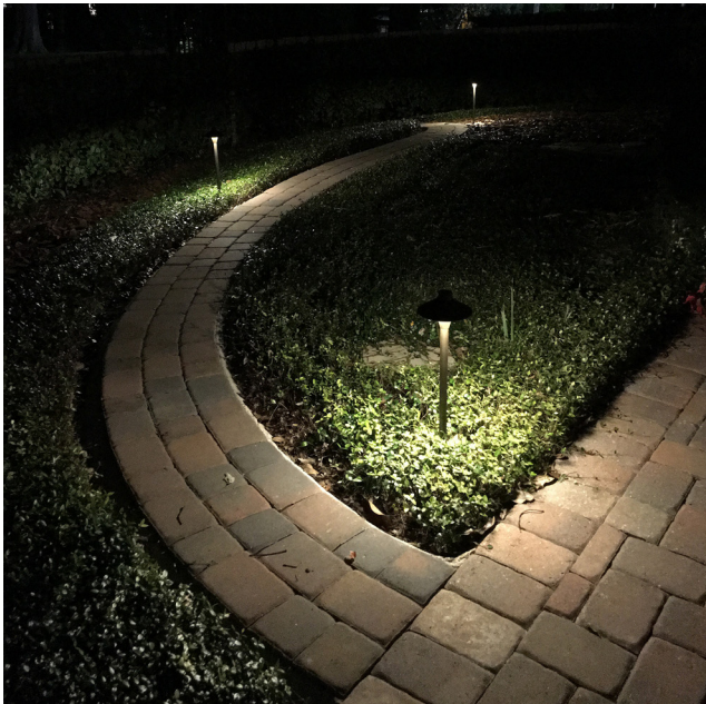
Low-height, fully shielded path lighting.
