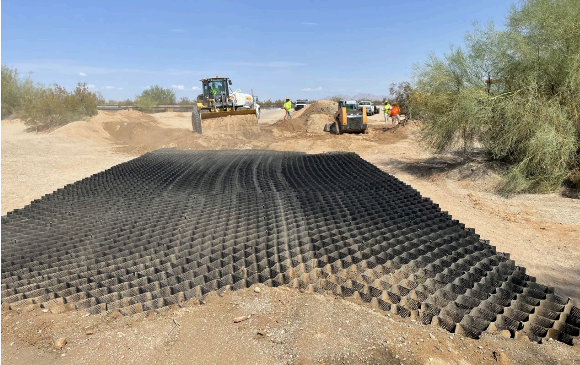
Photo: Installation of geo-webbing material under the Wash Road to prevent flash flood erosion in the Imperial Sand Dunes Recreation Area. Photo by BLM
