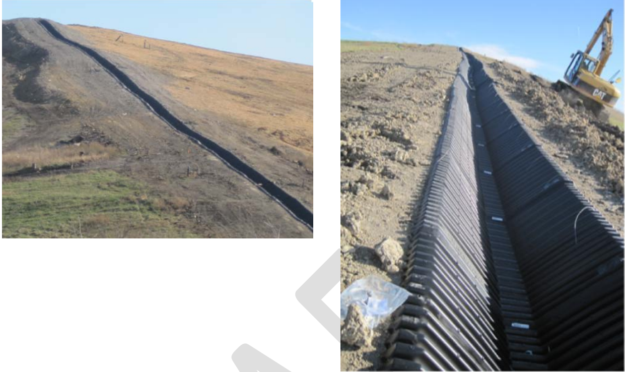
Figure 14 Example of a trapezoidal lining
