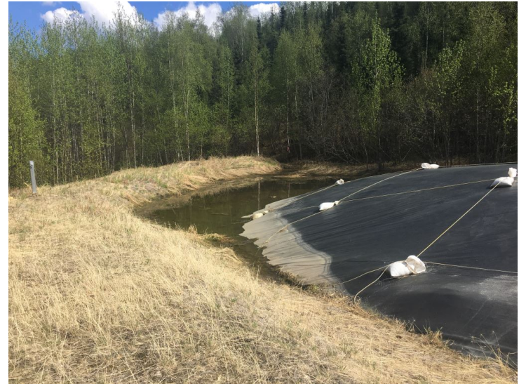
Photo 10: Flooding around settling pond.
