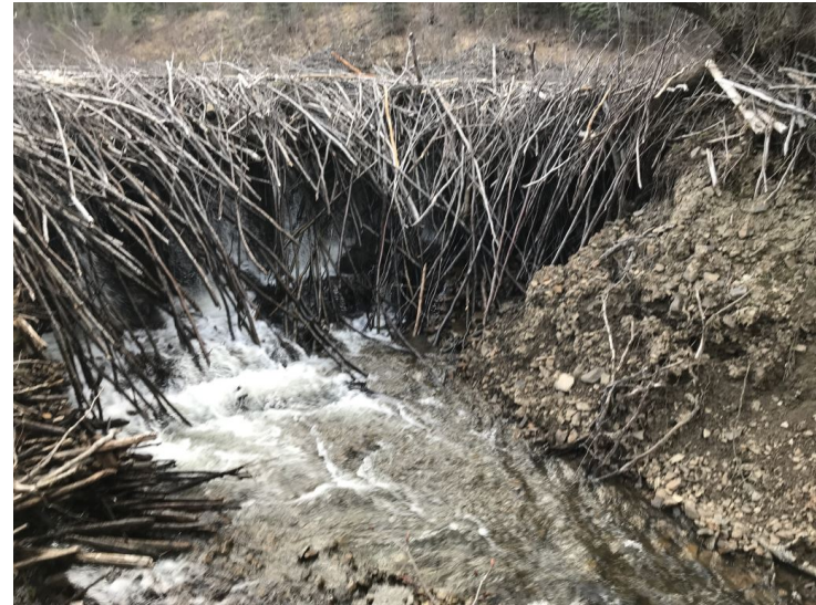
Photo 2: View upstream to breached beaver dam at Red Devil Creek Reservoir.
