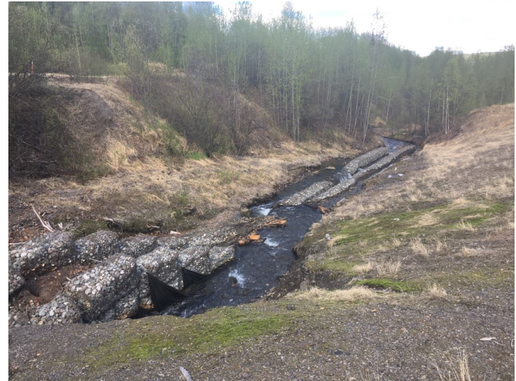
Photo 6: View downstream from the right bank of Red Devil Creek to the bypassed NTCRA.
