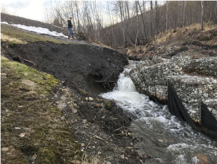
Photo 1: View upstream from right bank of Red Devil Creek during peak flow around breached gabions.
