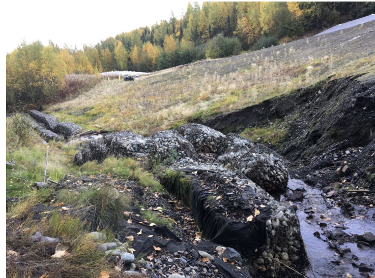
Photo 18: View downstream from uppermost extent of NTCRA gabions.
