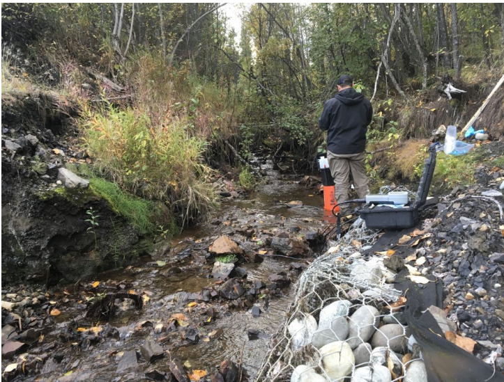
Photo 19: View upstream from the uppermost extent of NTCRA gabions.
