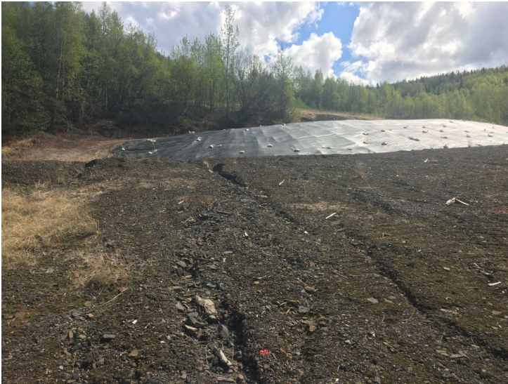
Photo 9: View upgradient from MW16 and MW17 to monofill.
