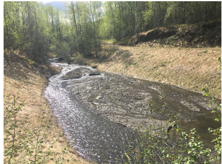
Photo 12: View upstream from right bank of Red Devil Creek to sediment settling pond.
