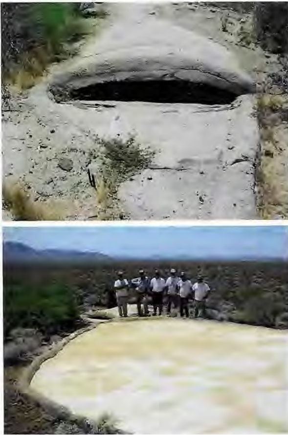
Figure 12. Rainwater catchment guzzler for wildlife at Mojave National Preserve, California; tortoises can become entrapped in guzzlers. Photos courtesy of Mojave National Preserve.
