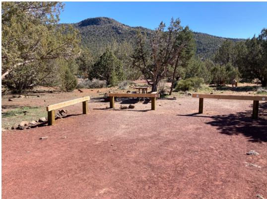
Barrier railing installed at Baker Dam Campground
