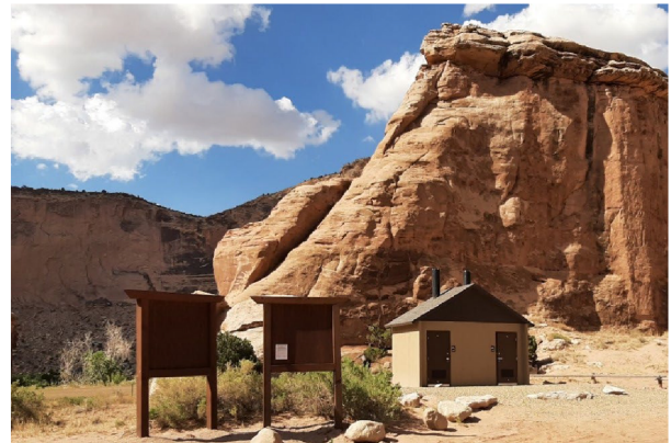
New Restroom and Kiosk in Buckhorn Draw
