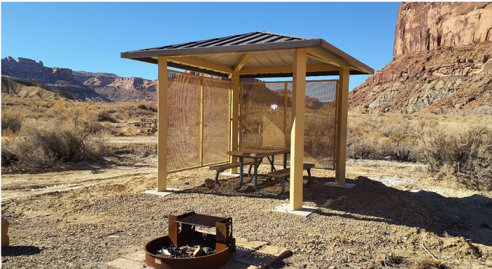
A New Shade Structure
