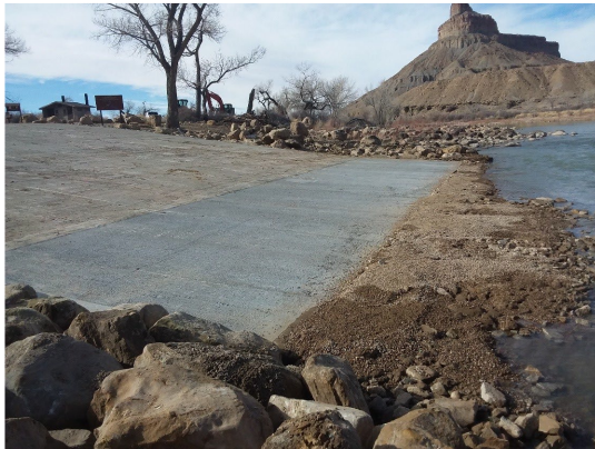
New Boat Ramp Extension
