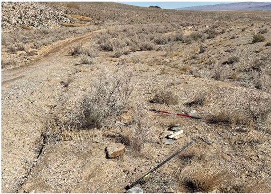
Installation of vehicle counters
