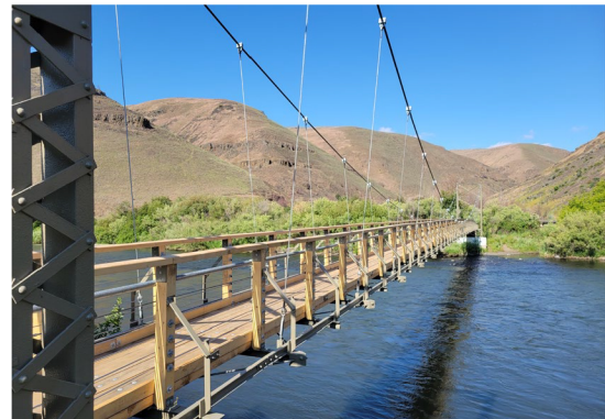
Completed Umtanum Bridge Improvements
