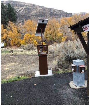
Install ROK unit at Umtanum recreation site
