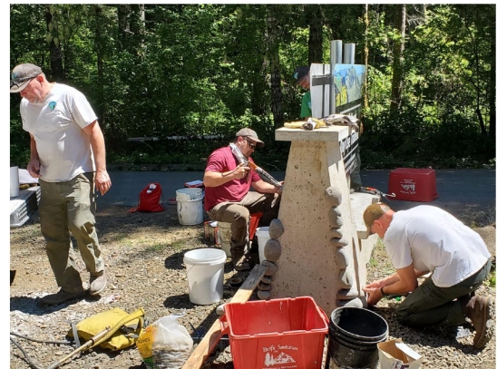
Recreation staff completing portal signs.
