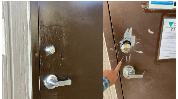
Replaced lock and handle.
