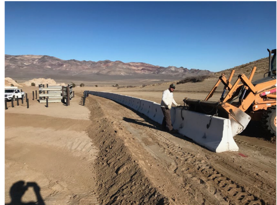
Completed bathroom pad and campsite delineation.
