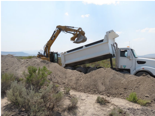
Road Maintenance within Soldier Meadows ACEC
