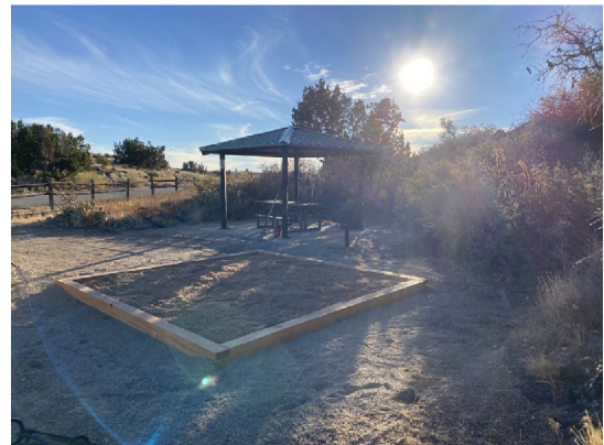
Tent Pad Replacement
