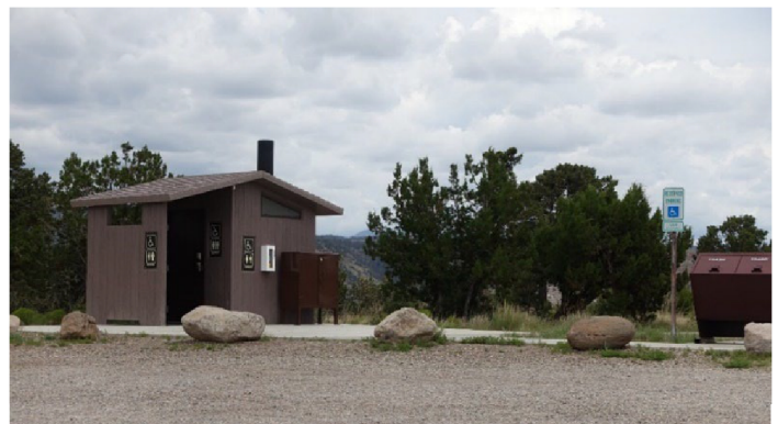
Picnic tables and vault toilets were painted
