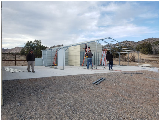
Contractors and Park Rangers installing Carport
