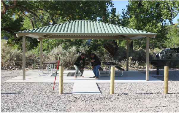
Improvements to the new MTB trailhead
