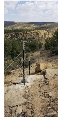
SMRA boundary fence replacement
